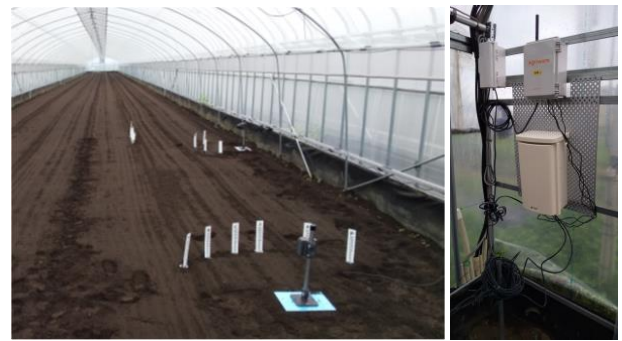
Fig.7 Installation of the system to a field of Kajitsudo Co., Ltd.
