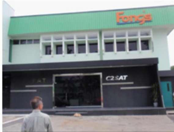
Figure4 Fong's Factory for VSAT antenna
